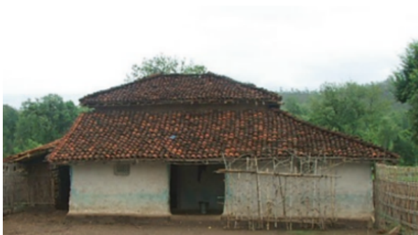
Figure 14. Open Entrance of a Traditional Mithila House
